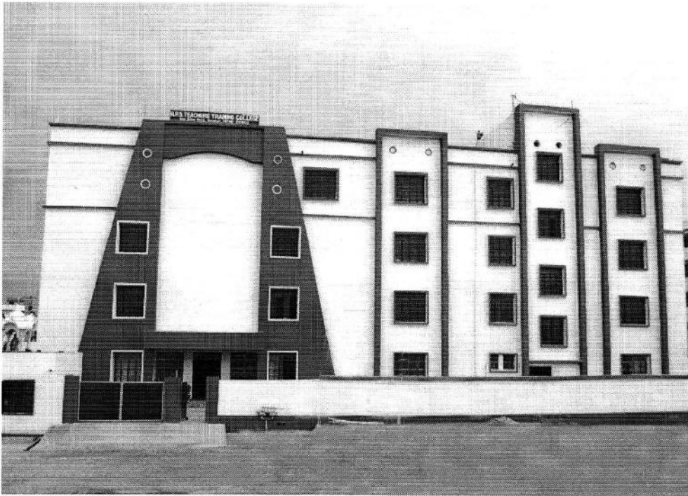
Rear view of the building
